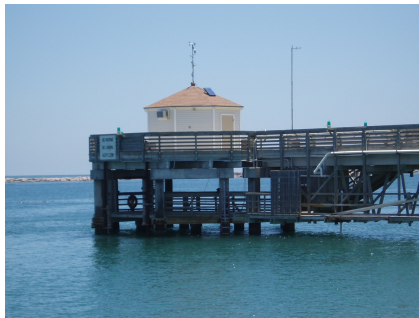
UT-MSI pier, Port Aransas, TX
